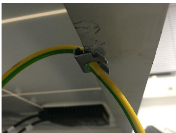
Figuur 7: Aardingsklem detail
